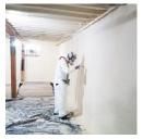
Concrete walls and floors can be sealed with foam.
